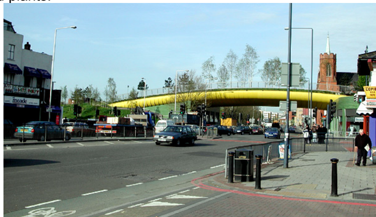
The Green Bridge
